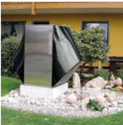
Air source heat pump, outdoor installation 15 kW
