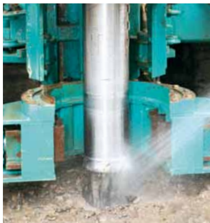
Drilling of vertical boreholes
